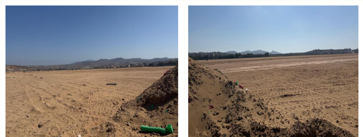
Figure 6-1: Photos from the Site
