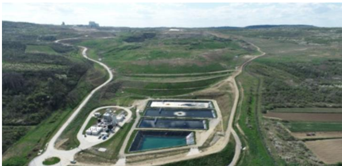
Vinca landfill after remediation. Source: Beo Čista Energija
