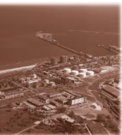
Ventspils port rail terminal project, Latvia
