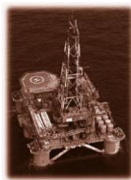
Chirag early oil project, Azerbaijan
